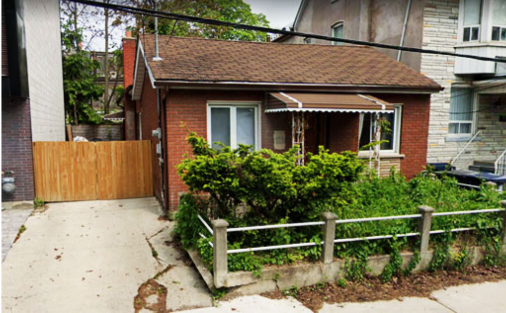
Figure 1: Boarded driveway across impugned easement 4
