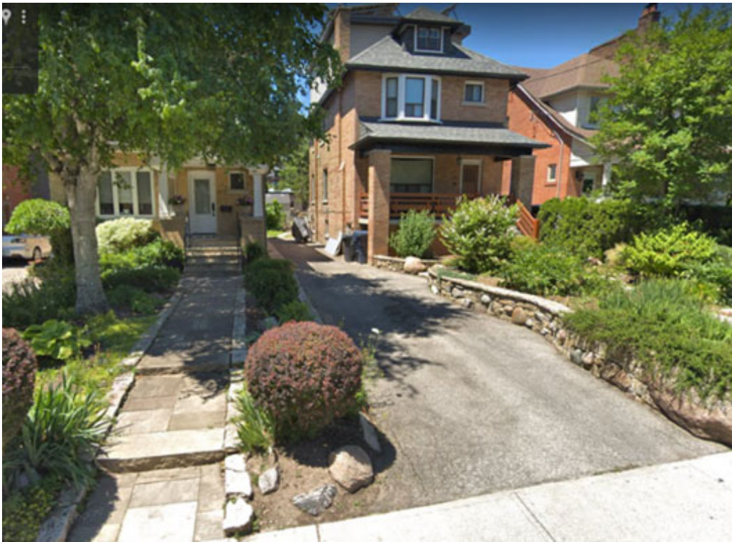
Figure 2: Street view looking west 5
