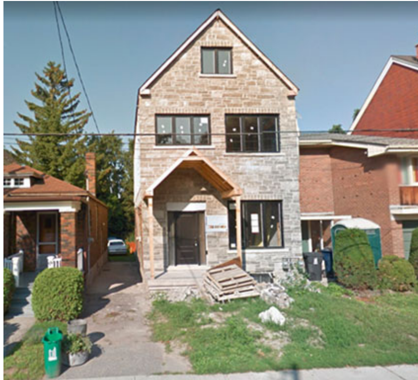
Figure 1: Home at No. 24 undergoing renovation and driveway to left 4
