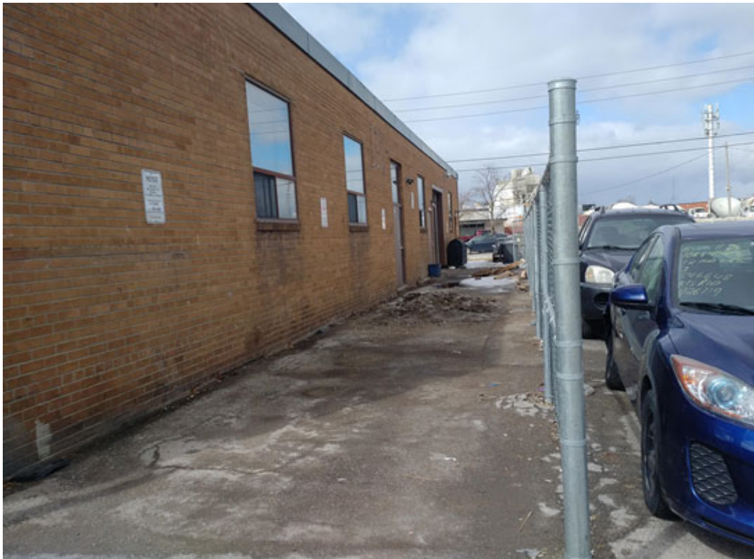
Figure 2. Driveway view of 35 Taber Road
