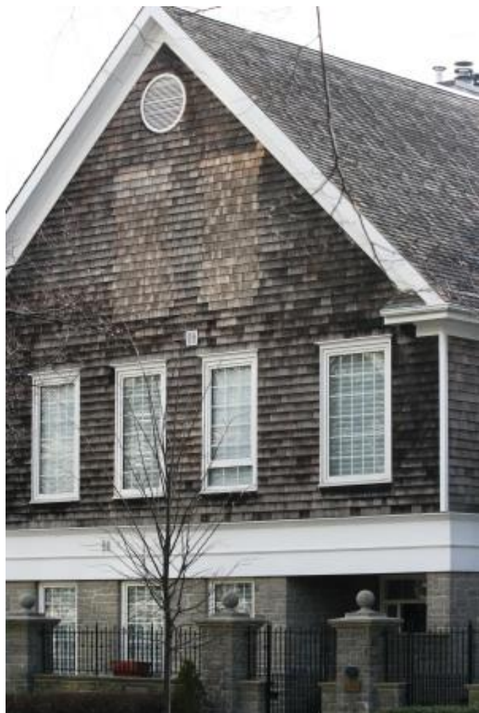
Figure 1: The former third floor had formed part of the living space
