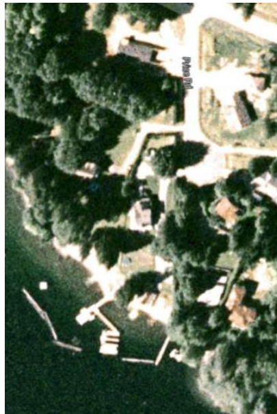
Figure 2: The dock structure with its protective log boom is readily apparent 7
